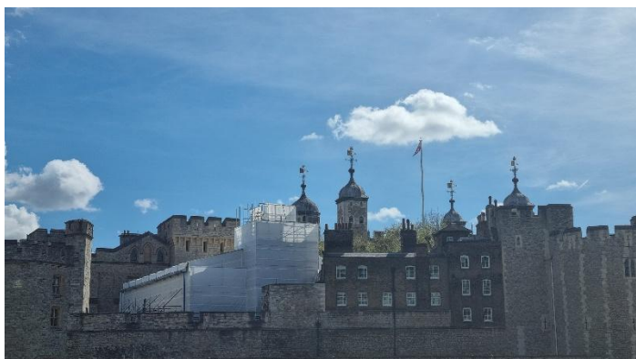
The scaffolding seen from Tower Hill
