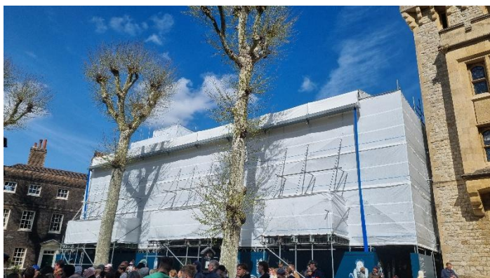
Scaffolding covering the exterior of the Chapel of St Peter ad Vincula
