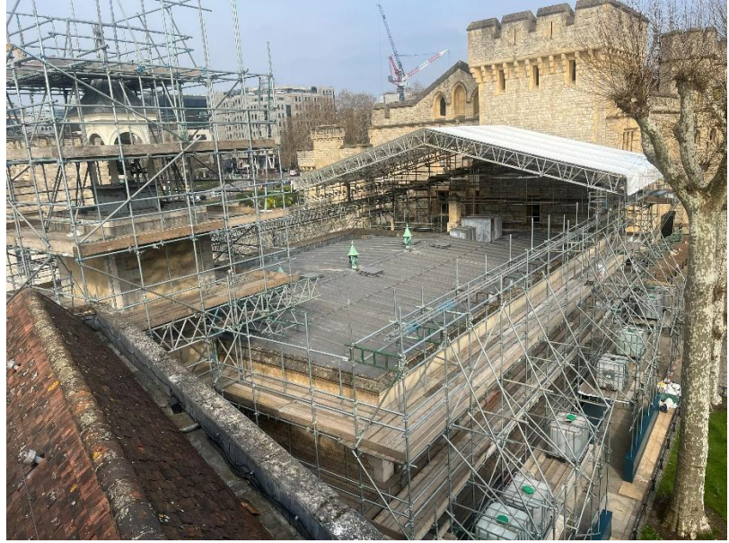
February – Scaffold build begins for the Chapel roof works.
